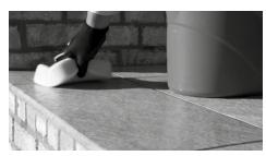
**PIC 5.** Removal of excess grout residues with hard brush.
