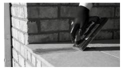
**PIC 1.** Fill joint with grout.
