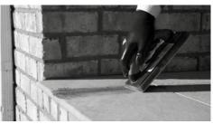
PIC 2. Remove excess grout with clean water.
